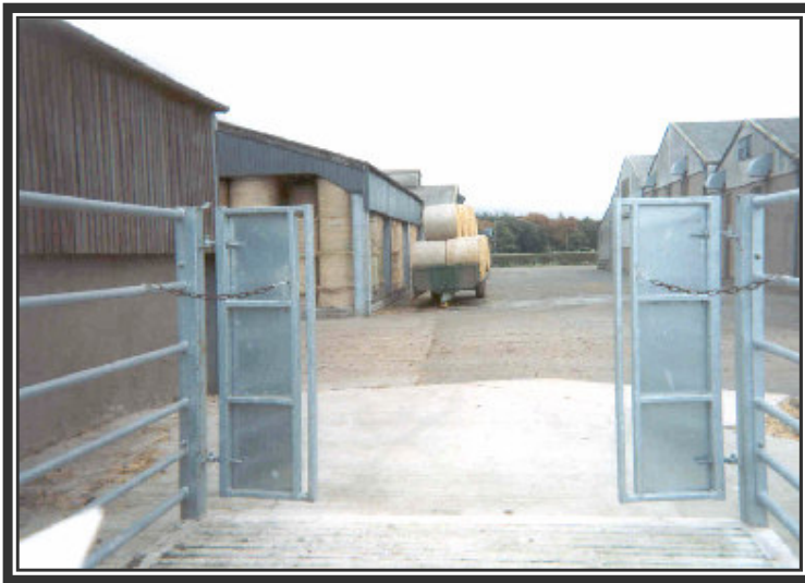
Figure 5.33.: These gates which are used to reduce the width of the ramp could impede the movement of animals whilst loading and cause bruising.
