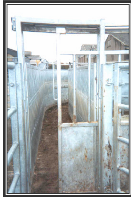
Figure 5.19.: A blocking gate which slides at 90° into the race.
