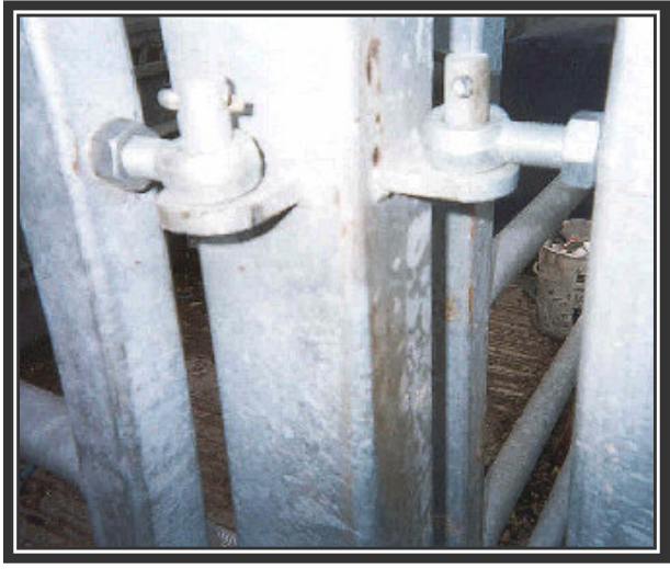
Figure 5.4.: The location of hinge pintles on square section posts should not prevent the full opening of the gate.
