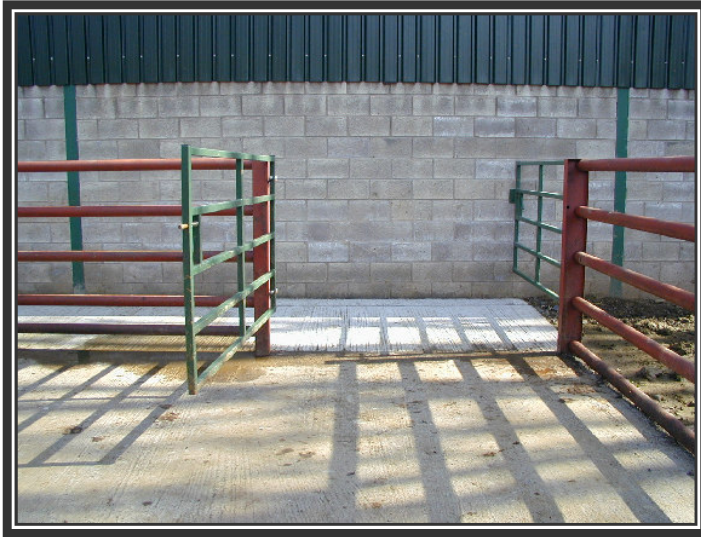
Figure 5.5.: The exit from this collecting / dispersal pen could be perceived as a dead end
